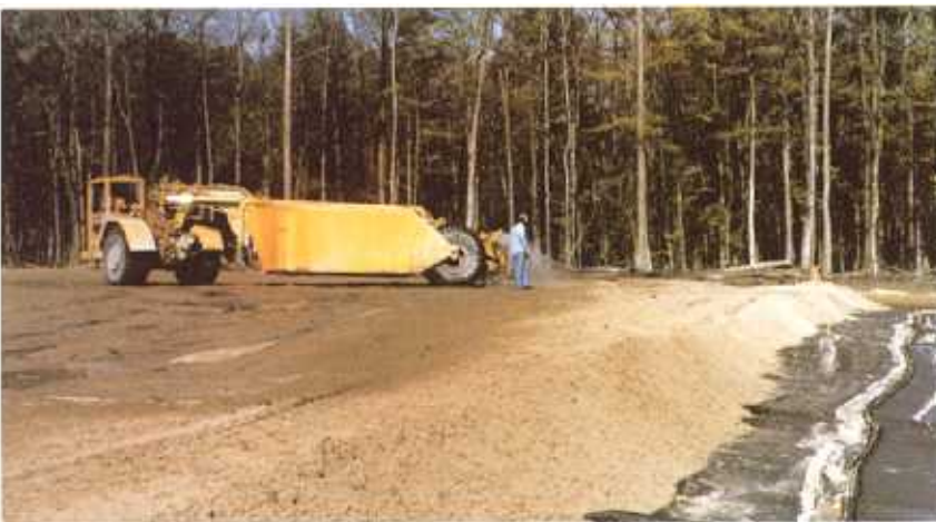
Embankment Fill ❖ Louisiana DOT D Test Project ❖ Morgan City, Louisiana
