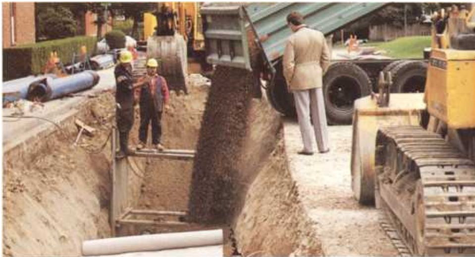
Calgary Pipeline ❖ Calgary, Canada Engineers: City of Calgary / Pildysh & Associates Consultants, Ltd.
