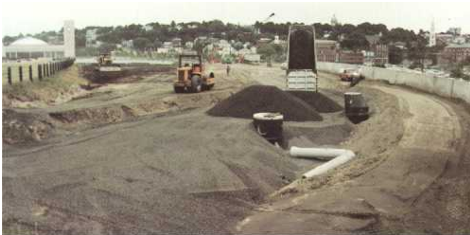
Retaining Wall Backfill ❖ Providence Rhode Island Engineer: C.E. Maguire Engineers, Mansfield, Mass.
