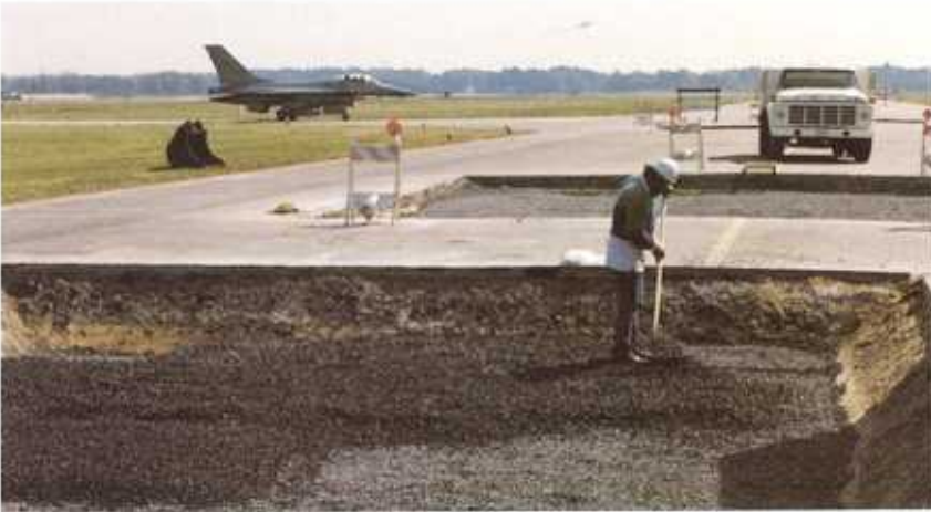
Runway Repair ❖ Norfolk Naval Air Station ❖ Norfolk, Virginia Engineer: Patton, Harris, Rust & Associates
